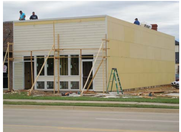
Office Building (MidTowne)
